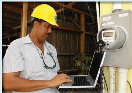
Employee inspecting meter as part of the System Losses Reduction Program.
