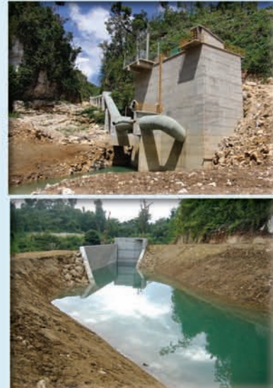
Hydro Maya's 3.4 MW power plant on the Rio Grande in the Toledo District came on line in February 2007.
